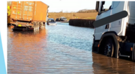
B645 at Stoneley flooded - December 2023
